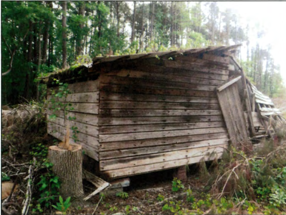
Figure 7. CD1481, Outbuilding 2 oblique of the south and west elevations, facing northeast.
