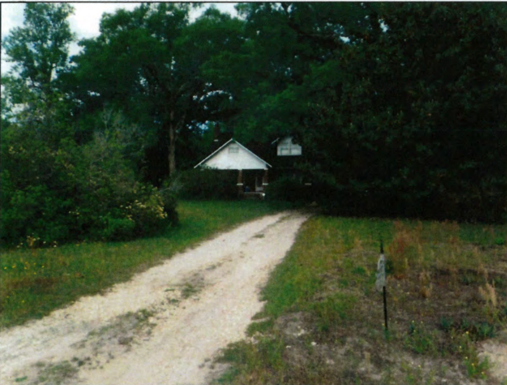
Figure 4. CD1481, dwelling south elevation, facing northwest.
