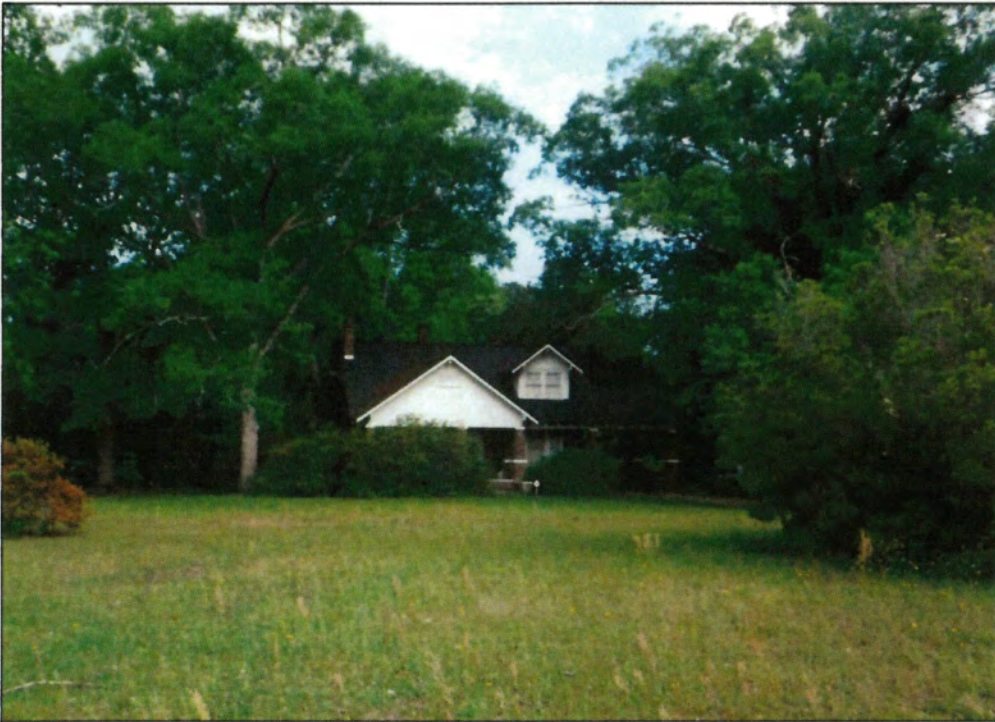
Figure 3. CD1481, dwelling south elevation, facing north.
