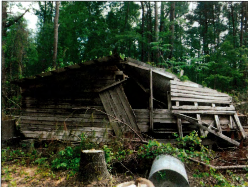
Figure 6. CD1481, Outbuilding 2 south elevation, facing north.
