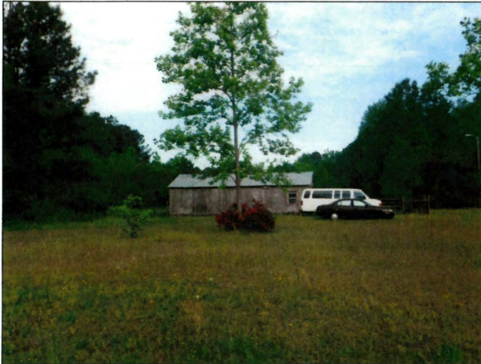
Figure 5. CD1481, Outbuilding 1 southeast elevation, facing northwest.
